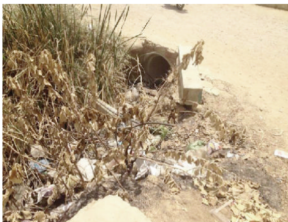
Choking of culverts at start point
