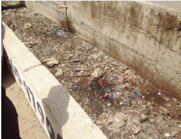
Solid waste deposition in unlined drains on both sides)
