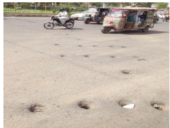
Openings for surface flow at KDA
