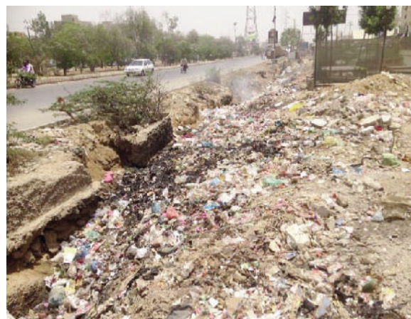
Choking of culverts at start point
