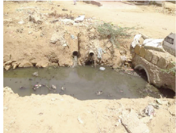
Choked Lined Drains at Powerhouse
