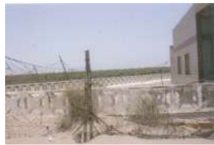
Illegal extension of a beach hut along with the erection of a wire net
