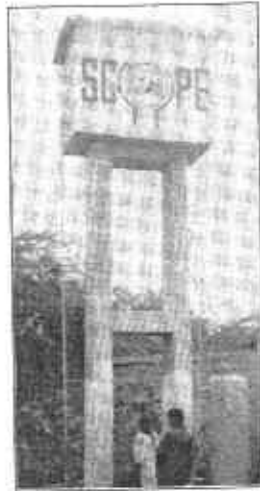
A view of a water purification plant installed by SCOPE.
